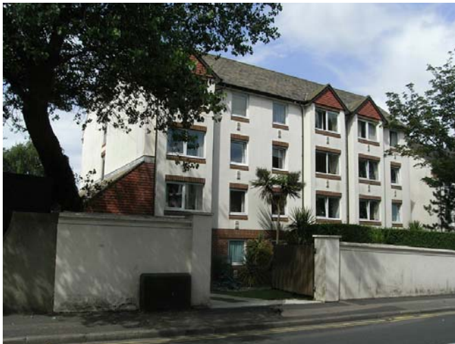
View of Homeless House
