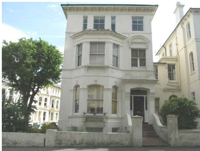
View of Dyke Road area
